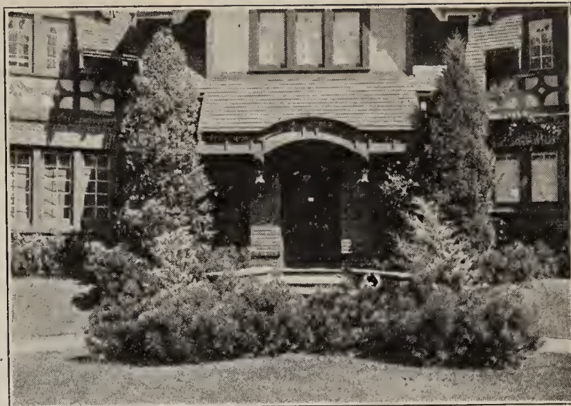
Note the Red cedar at the entrance and the mugho pine in the foreground
